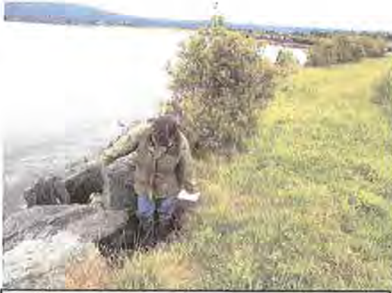
Photo 3 – View north showing eroded area proposed for repair along waterward top of bay front dike.
