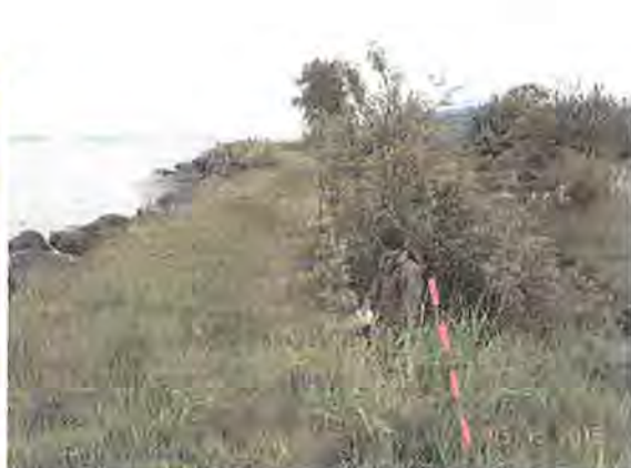
Photo 4 – View northwest showing portion of slump area (along dotted line) of slough dike proposed for restoration.
